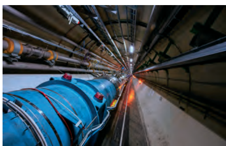
Section of the 27-km tunnel that houses the LHC particle accelerator at CERN
