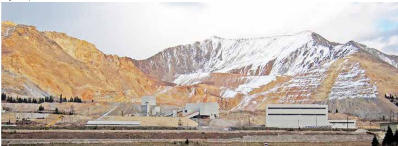
The molybdenum mine in Climax, Colorado, USA
