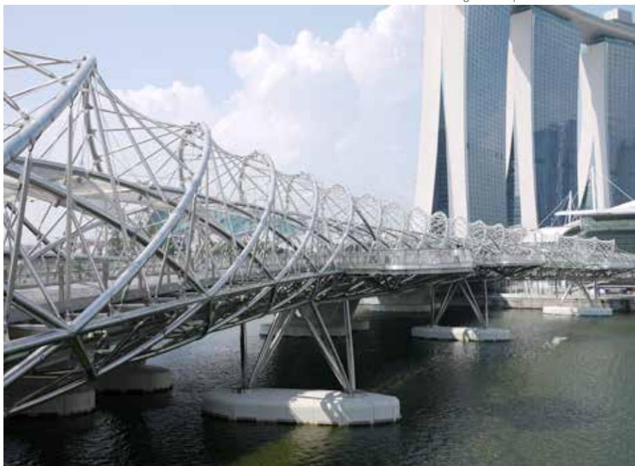
The helix bridge in Singapore, constructed using an alloy containing 2% molybdenum
