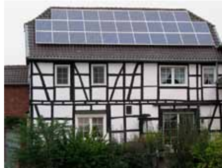
Photovoltaic array on a timber-framed house near Bonn, Germany
