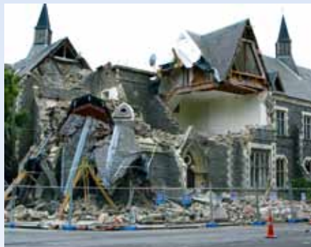
Damage caused by the 2011 earthquake in Christchurch, New Zealand
