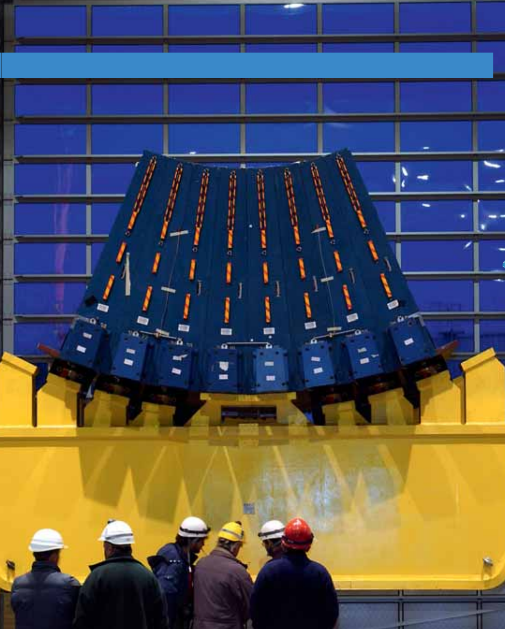
The tile calorimeter goes down into the ATLAS cavern
