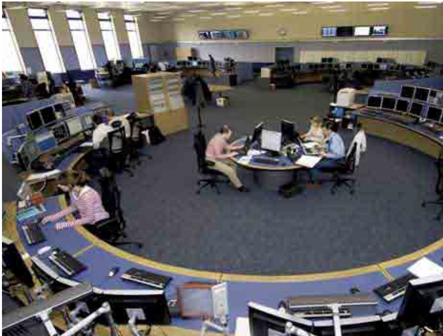
The control centre of the accelerators, the cryogenic distribution system and the technical infrastructure on the CERN site
