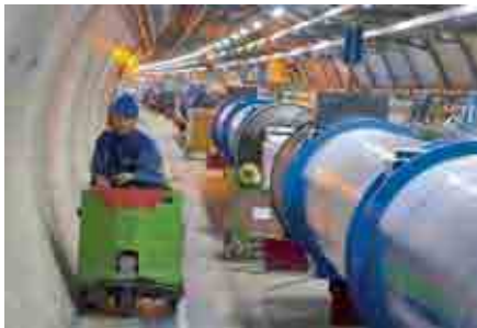
Technicians inspect the first magnets in the LHC tunnel
