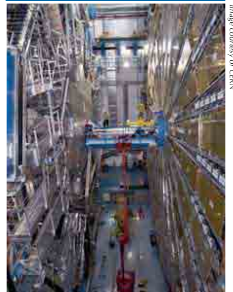
ATLAS beam pipe installation
