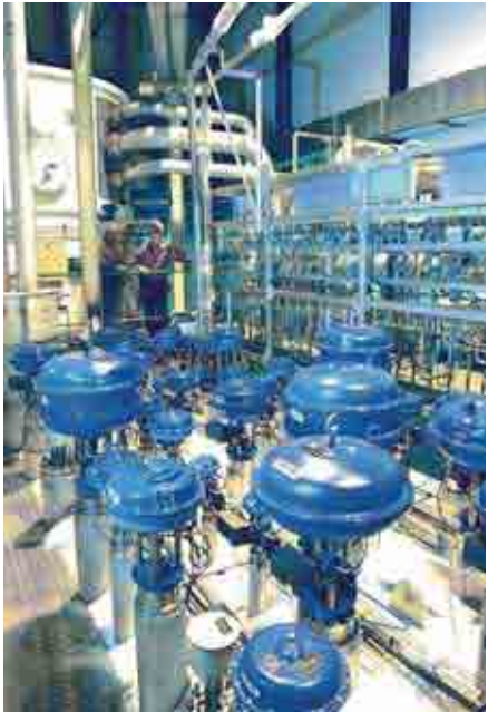
The cold boxes are major components of the LHC cryogenic system. This photo shows the top of the first cold boxes to be delivered to CERN
