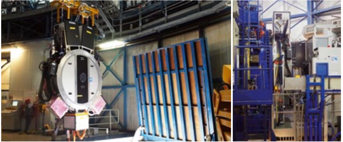
Figure 7. Left: GALACSI being hoisted through the azimuth hatch after transport from the Paranal New Integration Hall to UT4. Right: The very tight margin to manoeuvre this sensitive module between the Nasmyth acquisition and image rotator unit and the MUSE fore-optics can be seen.
