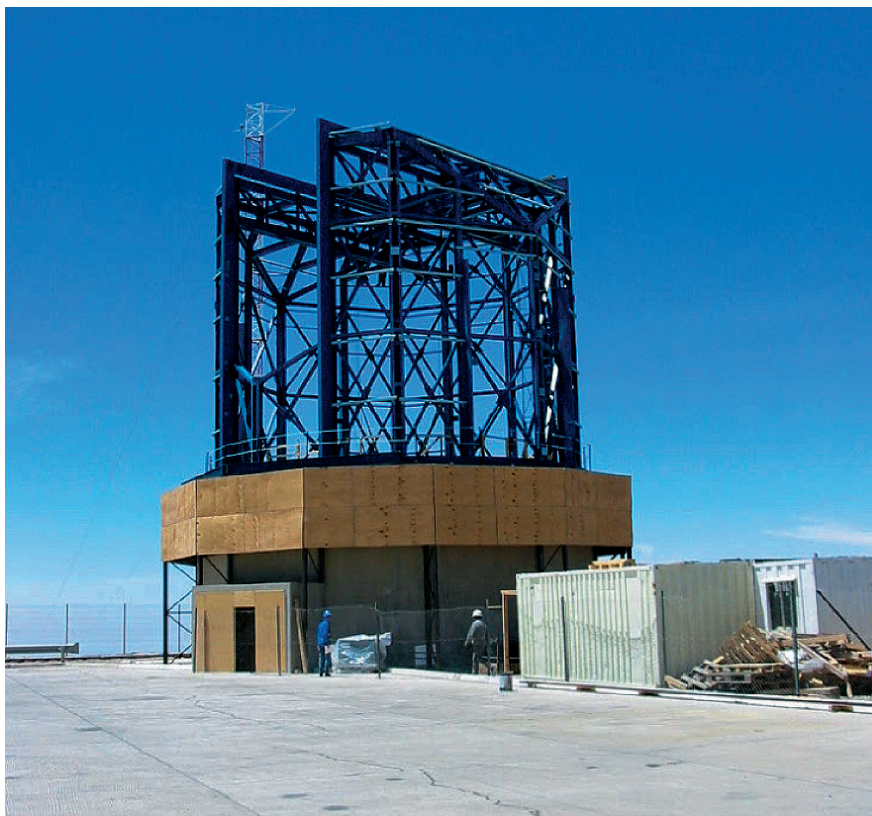
Figure 1: The VST enclosure taking shape at the edge of the Paranal platform.
