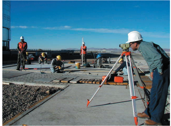
Figure 8: Installation of the AT interface devices inside each of the 30 observing stations at Paranal. A high-precision alignment method using theodolite and specific tools is used to reach a positioning accuracy below a millimetre and an arcminute.
