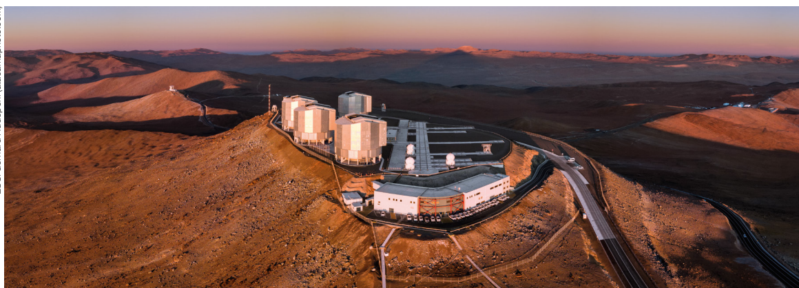
As dusk descends on ESO's Paranal Observatory, the four Unit Telescopes that comprise the Very Large Telescope (VLT) shine brightly, taking in the last rays of sunlight as they prepare for the night of work ahead.
