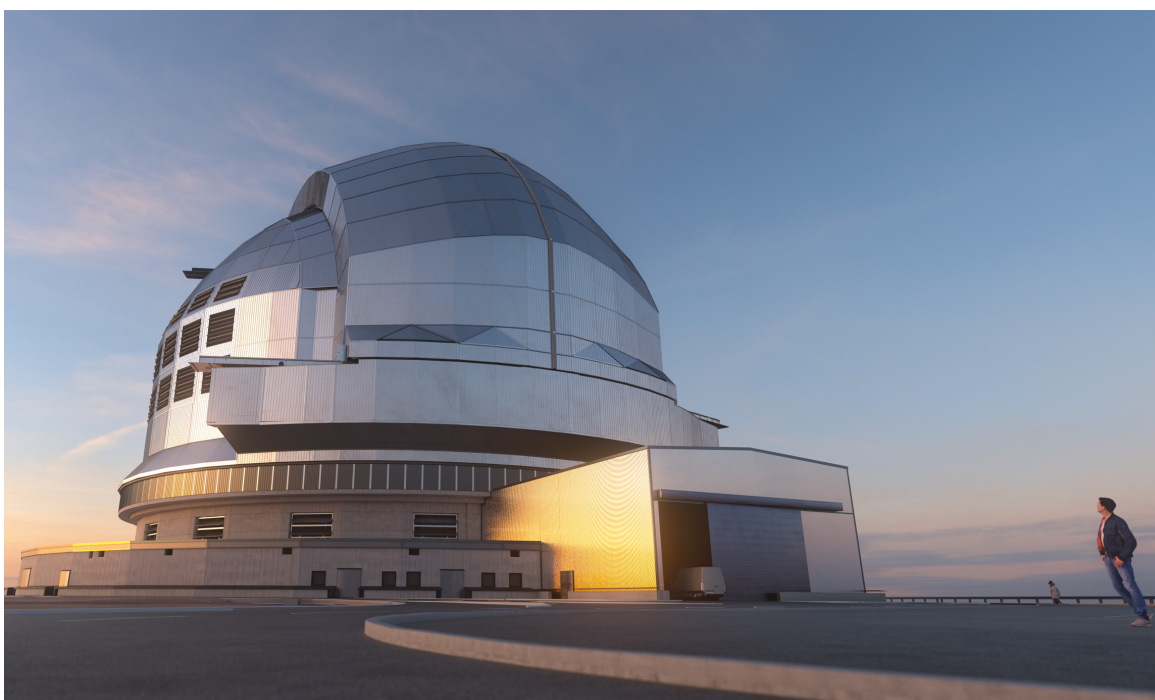
A huge structure is required to protect ESO's Extremely Large Telescope (ELT) from the elements. The telescope's structure and optical elements, including its giant 39-metre main mirror, will be housed in the largest telescope dome in the world, about 88 meters across, which is shown in this 3D rendering, along with the auxiliary building.
