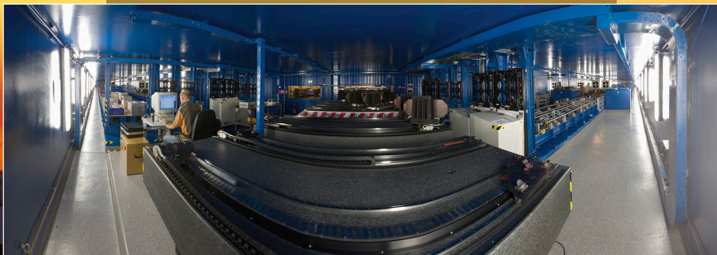
Panoramaoverblik over tunnelsystemet til Very Large Telescope Interferometer.
