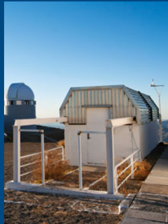
TAROT The sliding roof enclosure that holds the 25-centimetre TAROT (Télescope à Action Rapide pour les Objets Transitoires). It is a very fast-moving optical robotic telescope on La Silla that can provide fast and accurate positions of any quickly evolving events on the night sky within seconds.
