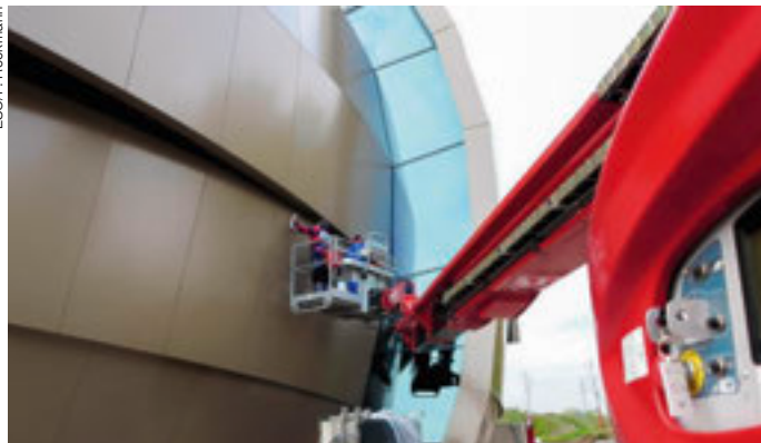
Cleaning the façade of the ESO Supernova Planetarium & Visitor Centre.
