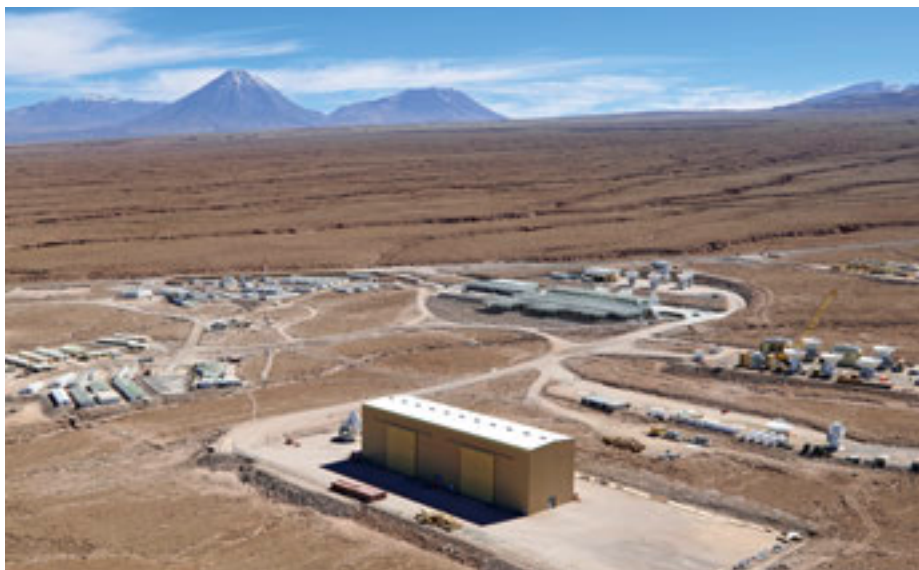
Aerial view of the OSF at 2900 metres above sea level. In the foreground is the antenna integration site where the antennas are assembled and tested by
