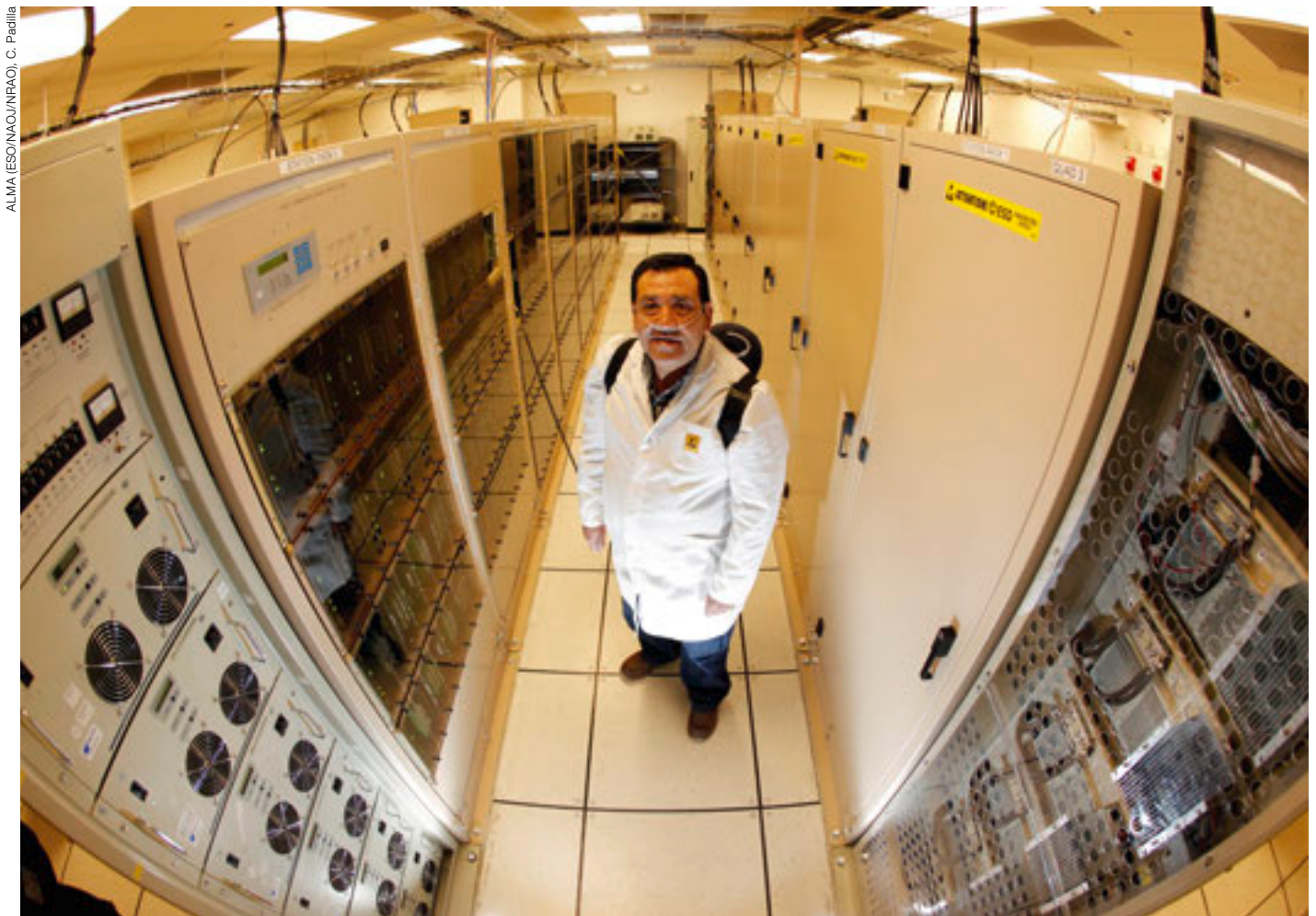
Correlator technician Juan Carlos Gatica with one of the most powerful supercomputers in the world, installed at ALMA AOS at 5000 metres above sea level, high in the Chilean Andes.
