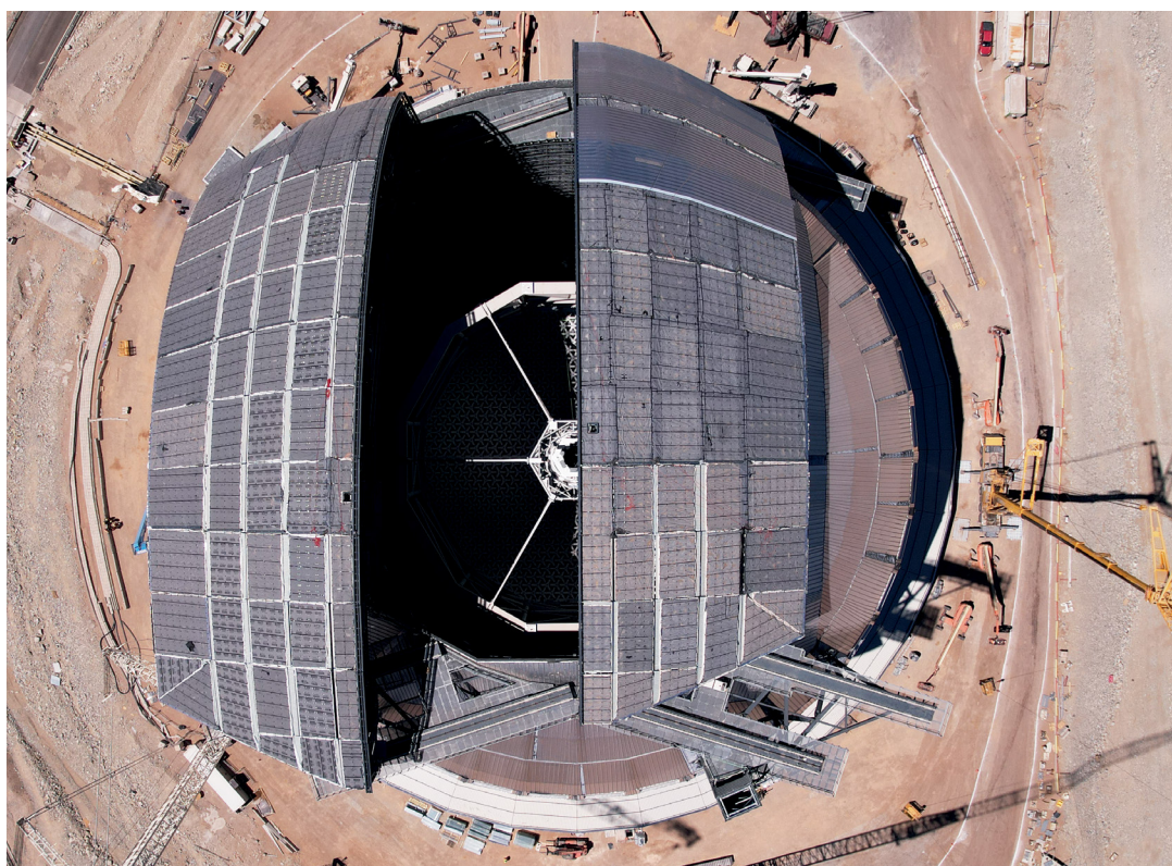
Aerial view of the ELT dome and main structure taken in November 2025.
