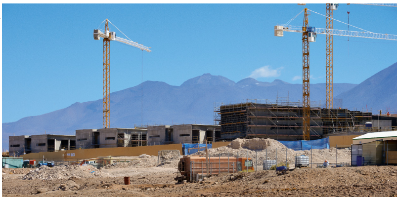
Construction of the ALMA Residencia started in February 2015 and was in an advanced state by the end of 2015.
