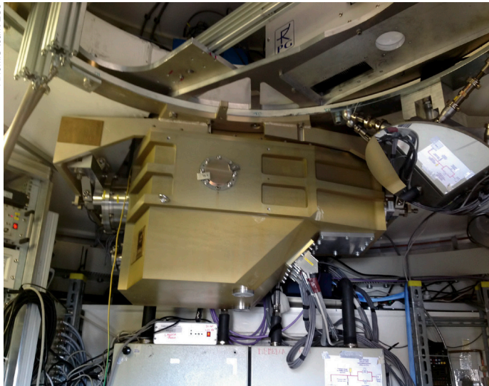
ArTeMiS instrument installed in the Cassegrain cabin of the APEX telescope.
