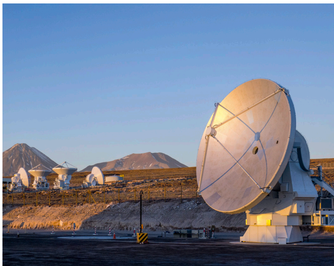
Final antenna delivered to ALMA.
