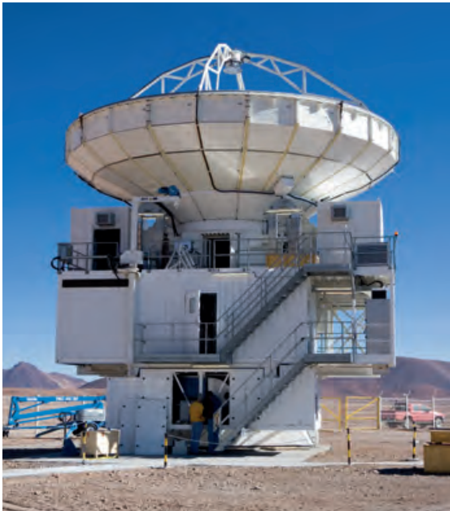
The APEX antenna. APEX is a collaboration between the Max-Planck-Institut für Radioastronomie (MPIfR), Onsala Space Observatory (OSO) and ESO.
