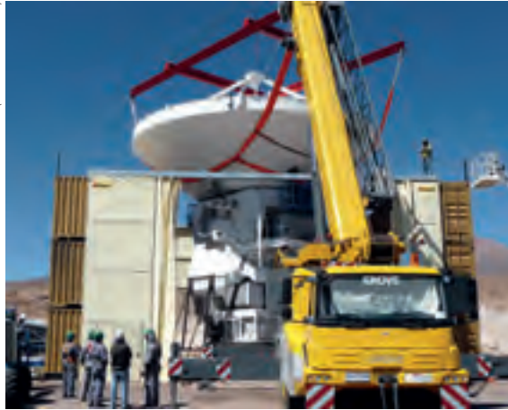
The first European antenna structure is being assembled.
