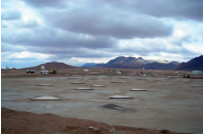
Antenna foundations for the ALMA central cluster.
