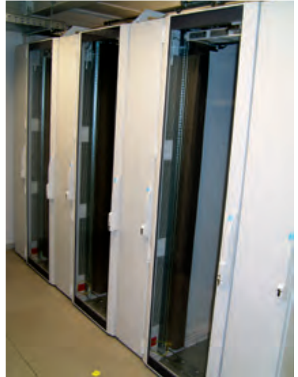
Actively cooled racks installed in the ESO Data Centre for the archive and database environment of the ALMA Regional Centre within the Data Management and Operations Division.
