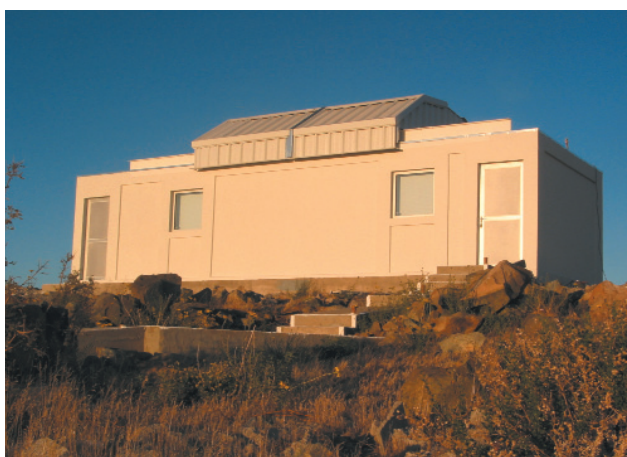
New building for the 60-cm IR robotic telescope REM at La Silla..
