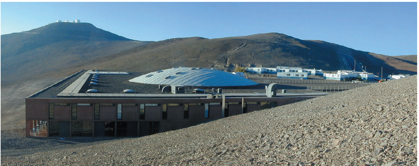
Exterior view of the Residencia, looking towards west. The linear construction used to fill the natural depression of the ground in this area is evident. The 35-m central dome protrudes from the "filled-in" valley.
