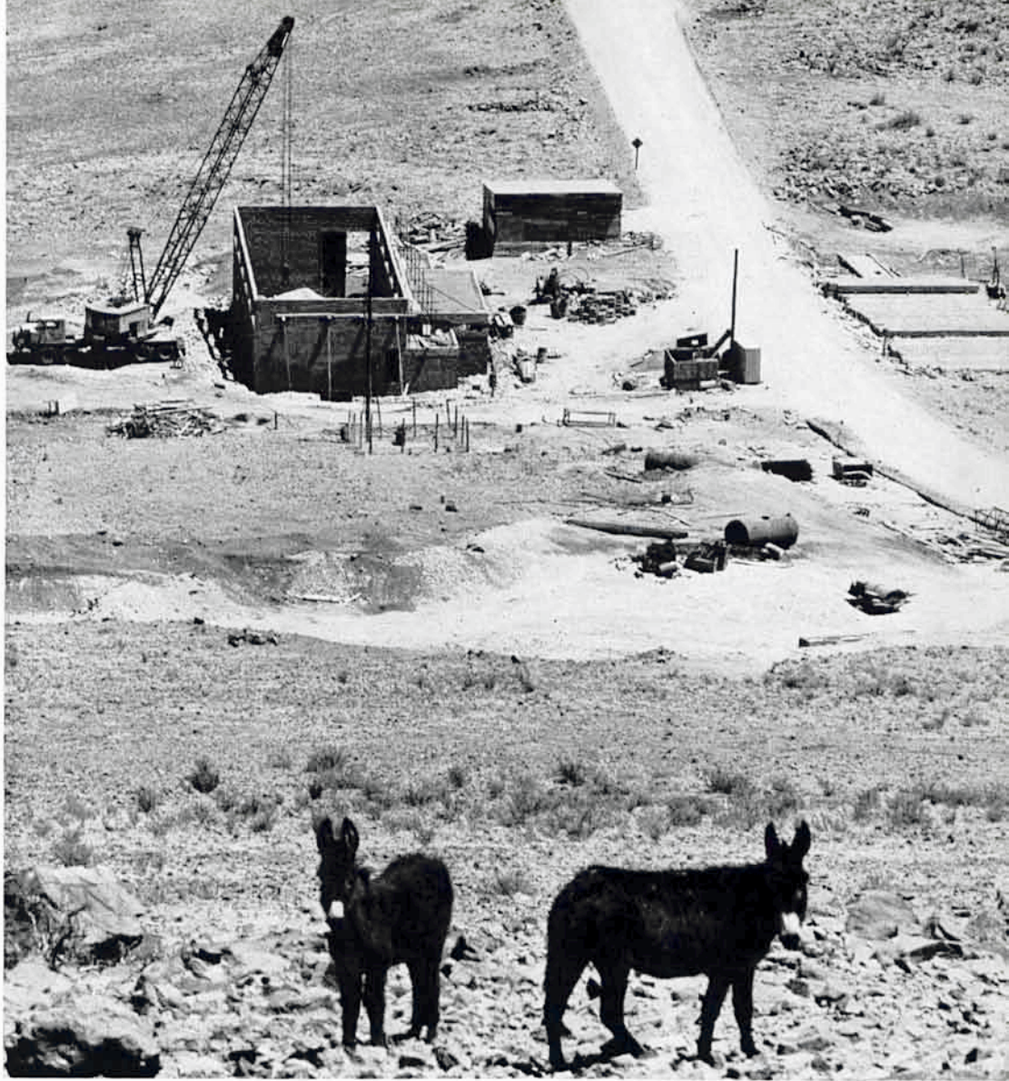
Construction of new power station.
